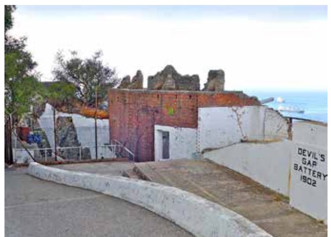
Devil's Gap Battery: the gorge of the southern of the two 6-inch guns, showing the rustic brickwork intended to disguise the battery's profile
